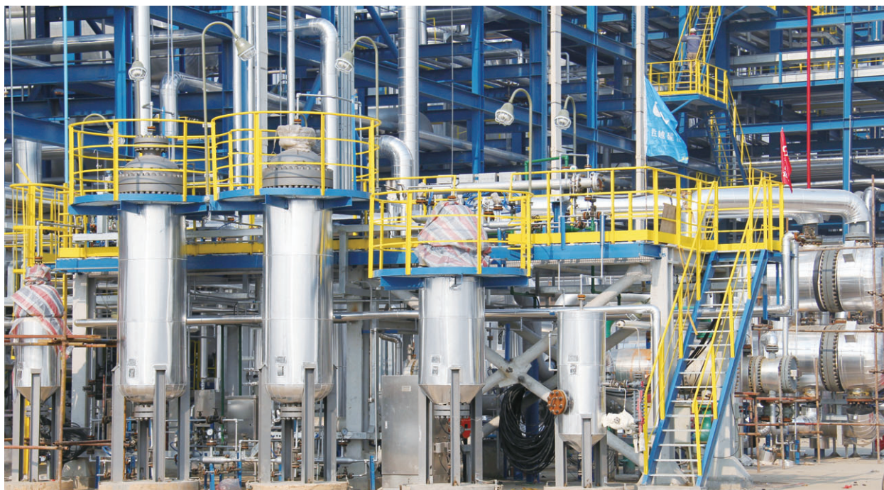
Hydrogen Oxidation Reactor (as at February 2015)
