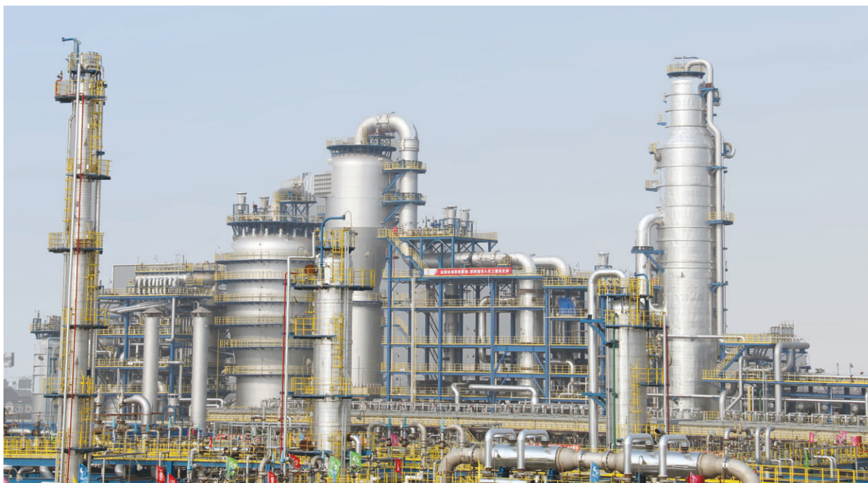
MTO's Reactors & Regenerator (as at February 2015)
